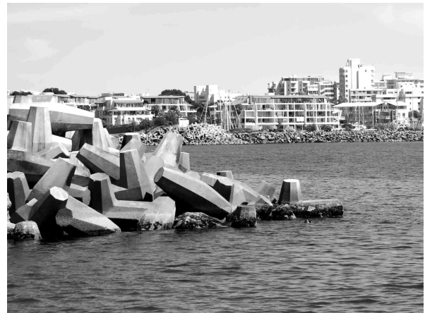
Figure 1: Dolosse protecting Cape Town's harbour
