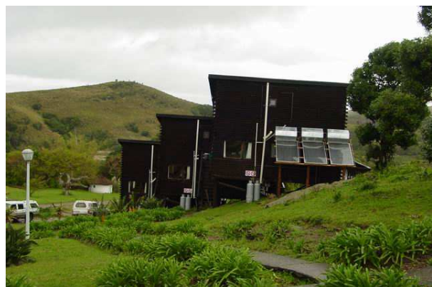
Figure 7: Solar water heaters and LPG bottles
