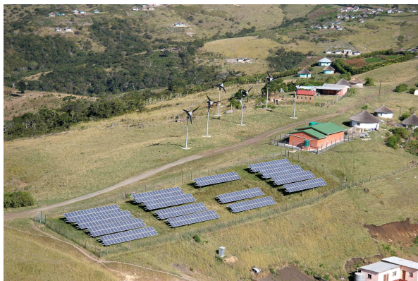
Figure 8: Lucingweni 86kW hybrid mini-grid
