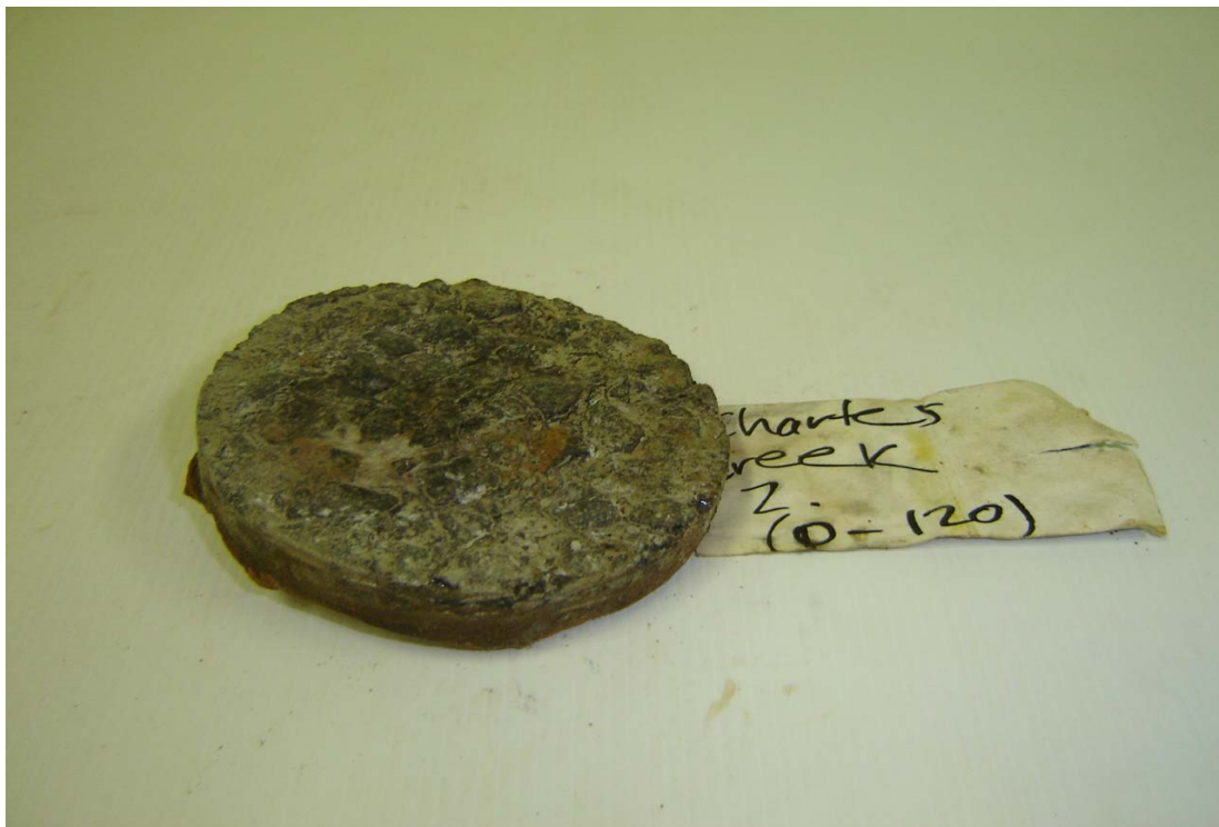
Photo 4 Core 2 on Charters Creek Road: Surfacing
