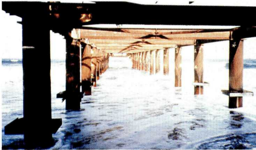
Temporary jetty for installation of pipeline (Photo: D.A Lord, UPE)
