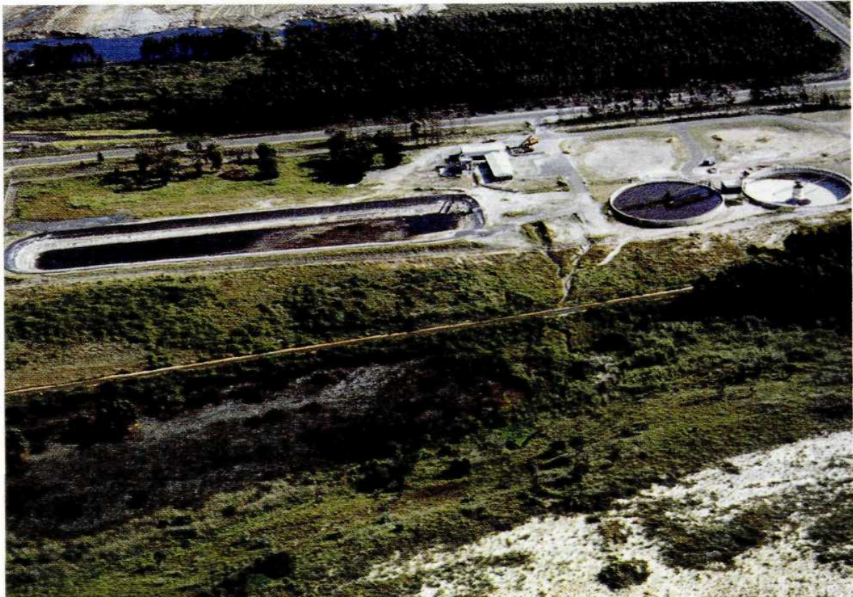
The Mondi Richards Bay effluent treatment plant, showing the twin clarifiers and the reserve holding dam (Photo: supplied by Mondi Pulp Mills)
