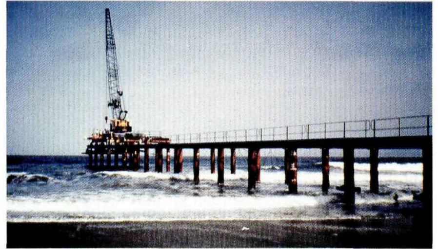
Temporary jetty through surfzone (Photo: D.A Lord, UPE)
