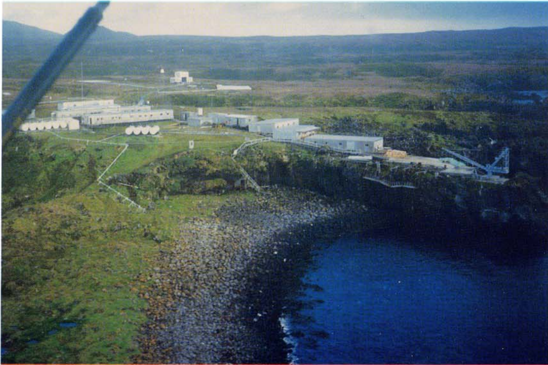
FIGURE 1.3 Aerial view of the Base Station on Marion Island. The central complex comprises living quarters, power plant and store rooms. In the middle background are helicopter landing pads and the radiosonde balloon release and tracking hut. Boulder Beach of Transvaal Cove in the centre foreground, Gentoo Lake in the left foreground, and Gunners' Point with the cargo hoist centre right.
