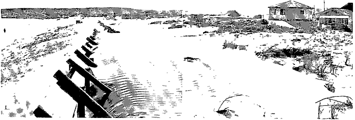
PLATE 133. Slat-fence erected at Stilbaai to protect beach houses from becoming smothered by drift sand. A new littoral dune has been formed but sand drift continues as there has been no follow-up operation to stabilize the sand. Cape south coast.
