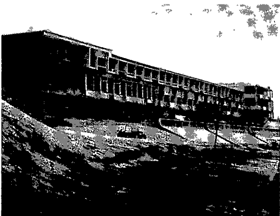
PLATE 98. Playing King Canute with a major material investment. Beach hotel built in the littoral on sand. Despite the concrete apron it has undergone repeated massive damage from waves. Xai-Xai area of Limpopo Coast, south Mocambique.
