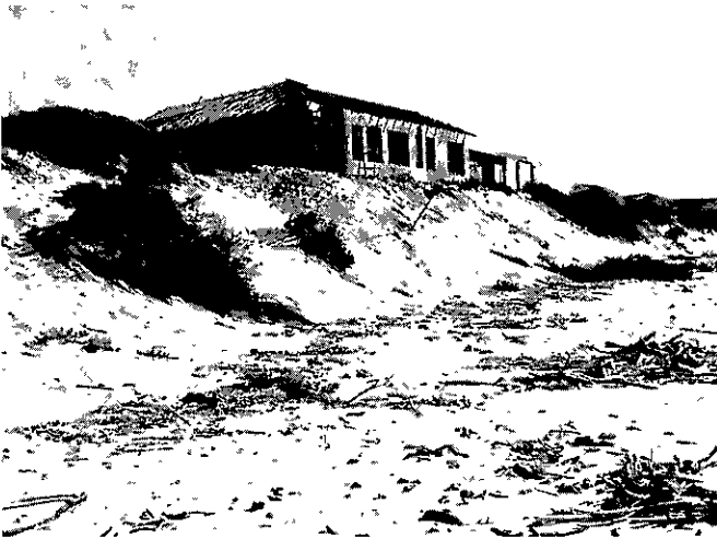
PLATE 136. Erection of sumptuous holiday houses at the coast in the ephemeral strand plant zone. Albatross area of Jeffreys Bay, St Francis Bay.
