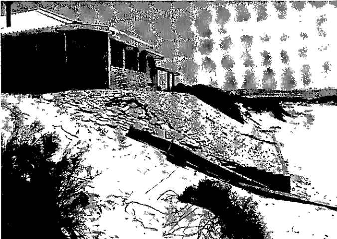
PLATE 137. The same house with newly completed, rock-paved, concrete apron already under high tide wave attack (undermining and cracking). Note cliffed duneshore in background.
