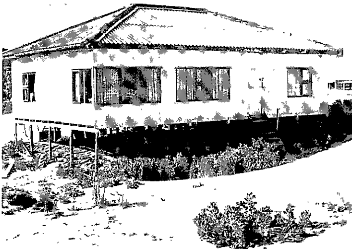
PLATE 134. Beach house supported by stilts as dune sand was scoured out from beneath the foundations to form a typical wind scour hollow associated with solid objects in dunes.
