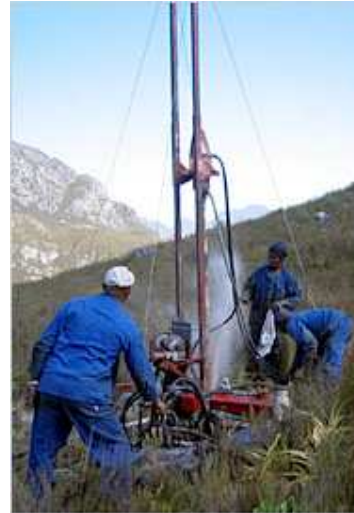
Drilling in the Table Mountain Group aquifer
