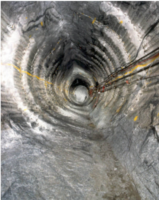
Figure 12 Inclined dog earring in a tunnel illustrating an inclined in situ stress direction (photograph provided by Dr C D Martin)
