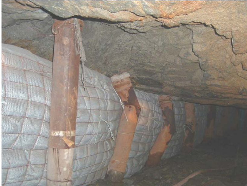
Figure 3.3.2 Backfill in the E9 panel.
