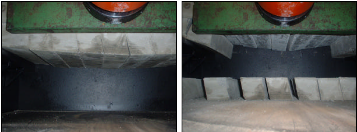
Figure 30. Underside of the beam before and after fallout
