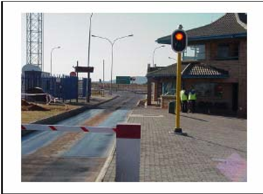
Figure 3: Multi - Deck Static Weighbridge scale (permanent installation) at the N3-TCC
