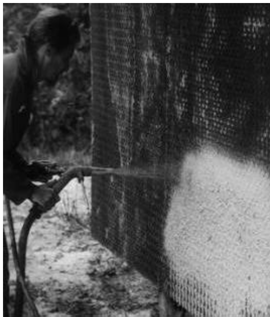
Figure 16. Spray application of Evertherm to a test panel.
