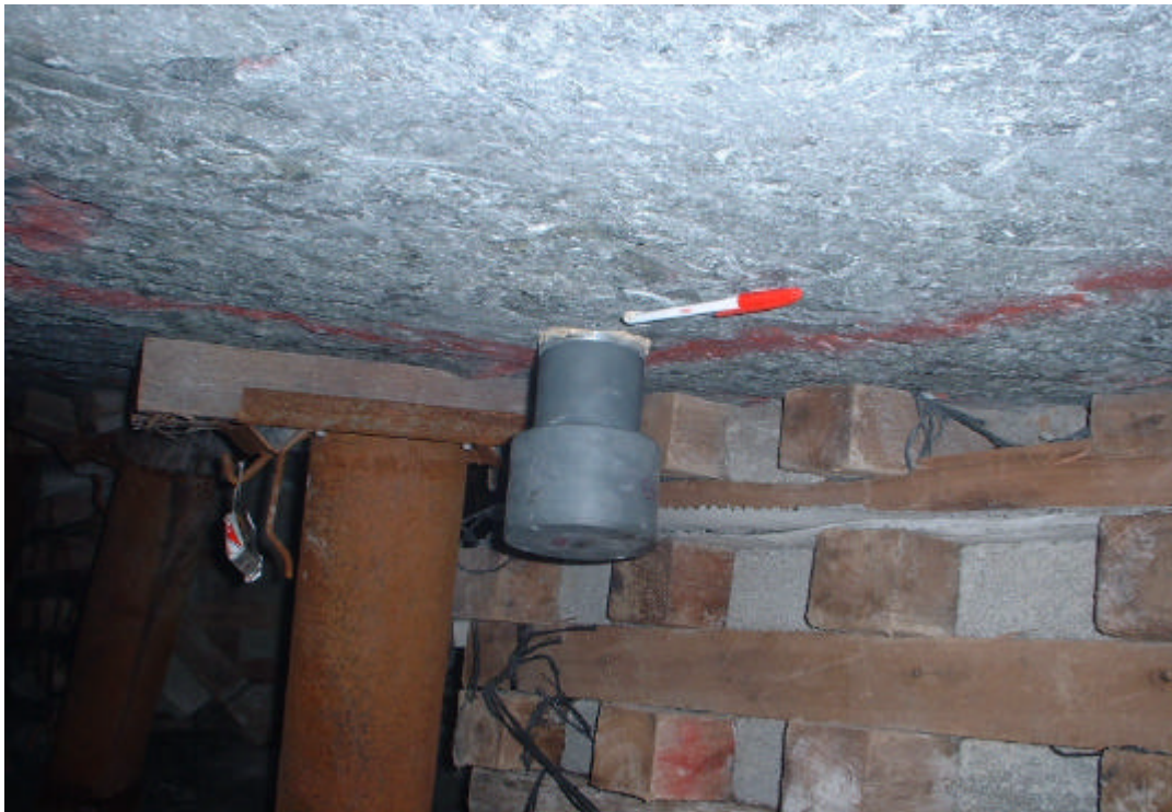
Figure 2.8 Underground site in Kloof gold mine illustrating the installation of the PVD
