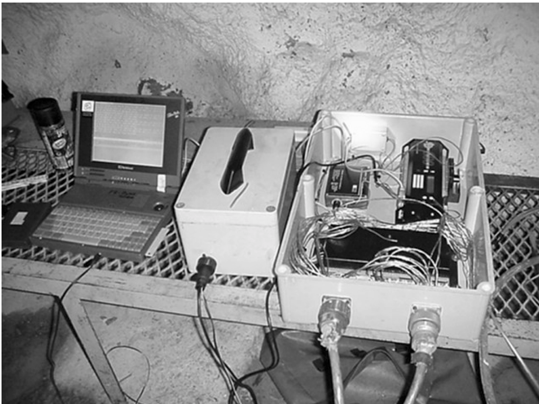
Figure 5.2.6 Data acquisition system in use on the site at Impala platinum mine
