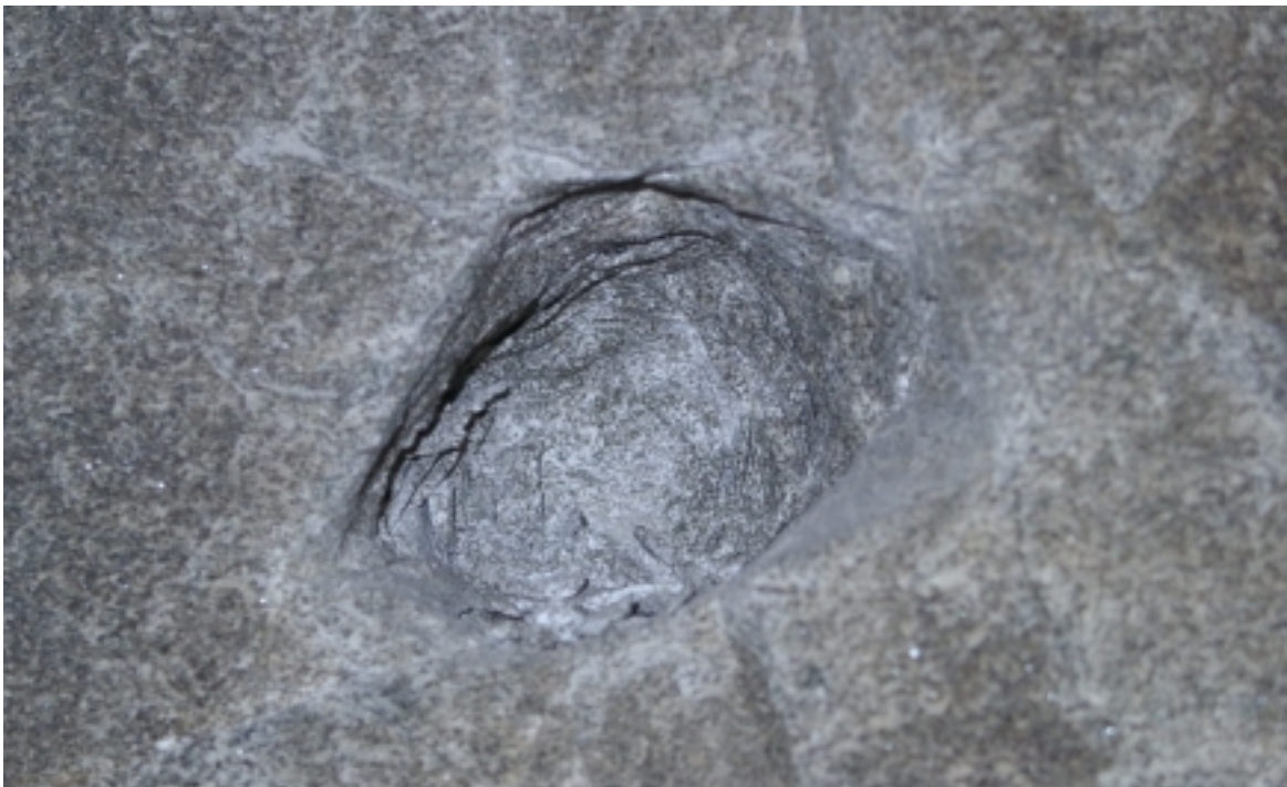
Figure 6.1.3 Photograph of borehole breakout in the vicinity of the tunnel
