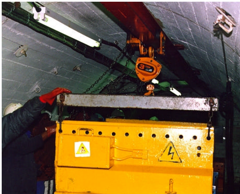
Figure 4.2.5.1: Battery pack lifting operation
