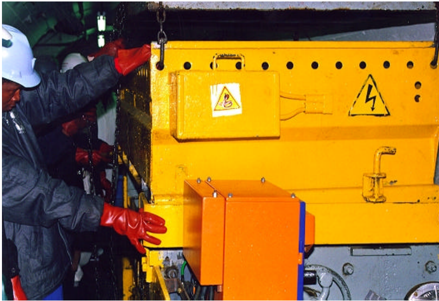
Figure 4.2.5.2: Battery pack lowering operation
