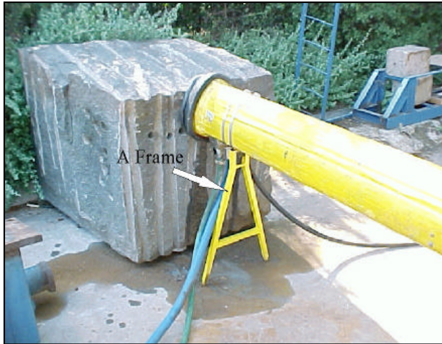
Figure 4-5 A-frame support of the drill at the rock face
