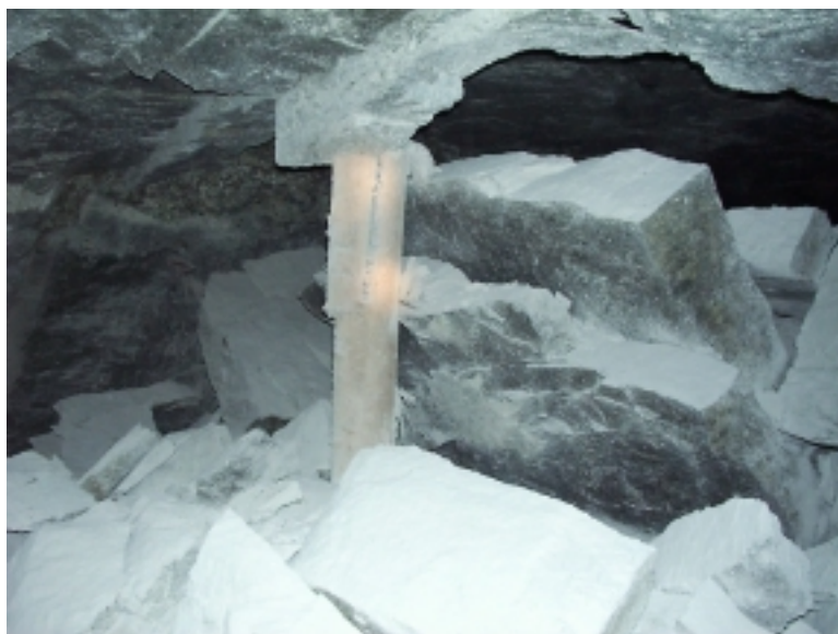
Figure 2.3.7 Photograph showing blocks fallen around a support element.
