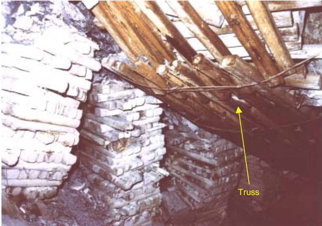
Figure 4.38 – On-reef trackless roadway supported with trusses and cribbing (before rockburst)
