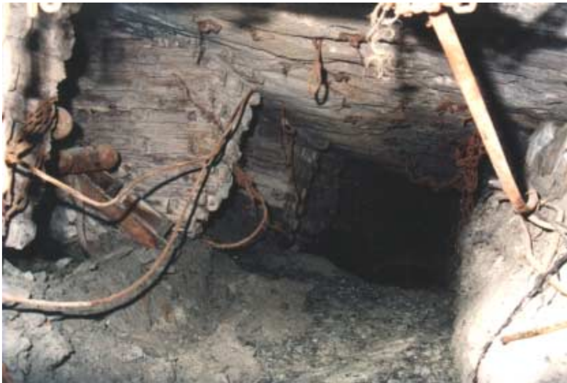
Figure 4. 35 - VCR footwall lifted gully – good hangingwall conditions
