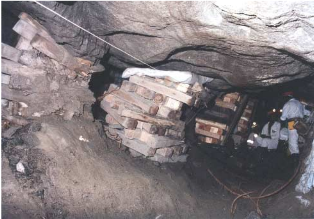
Figure 4.50 – Gully shoulder and hangingwall unevenness results in uneven compression of pack and its eventual disintegration
