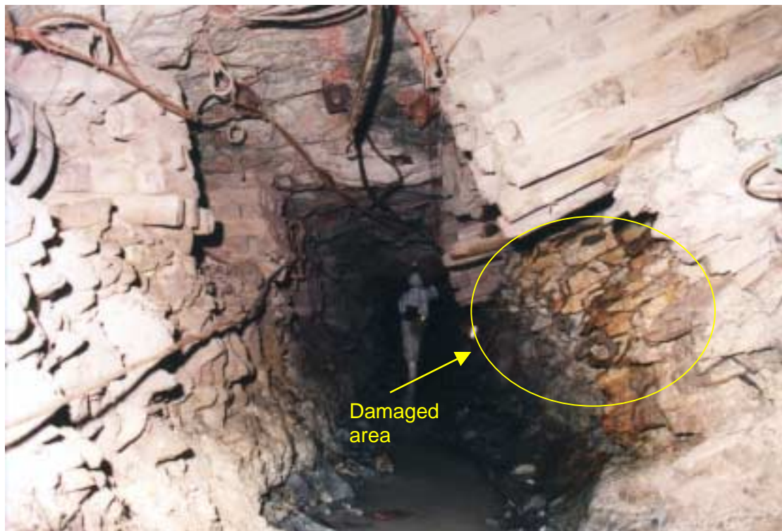
Figure 4.48 – Scraper erodes up dip sidewall of gully beneath packs
