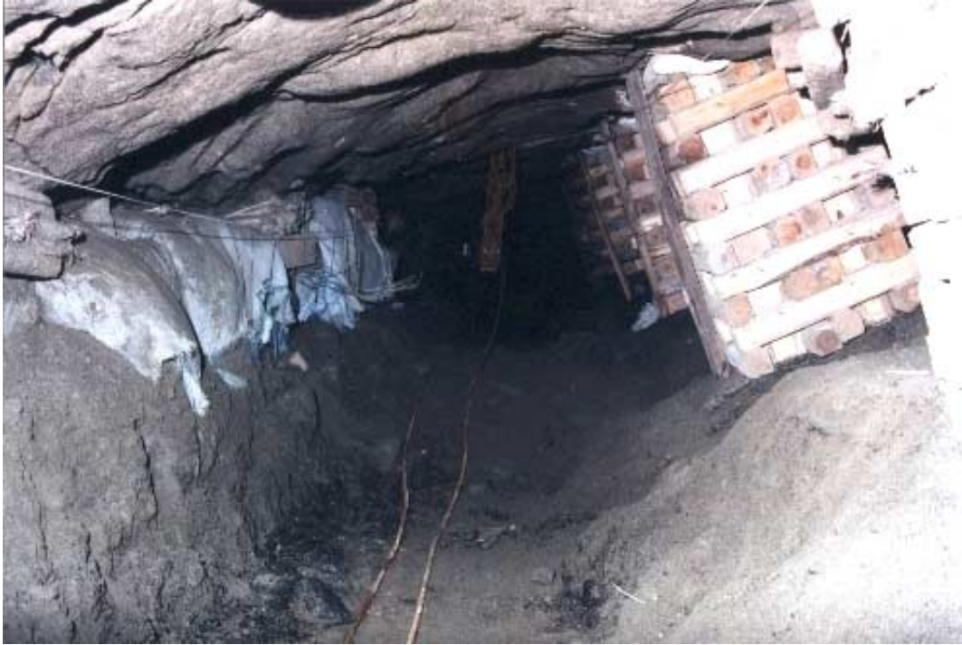
Figure 4.24 – Conditions along a footwall lifted gully on the Merensky Reef at 2000m. Note backfill installed on the down dip side
