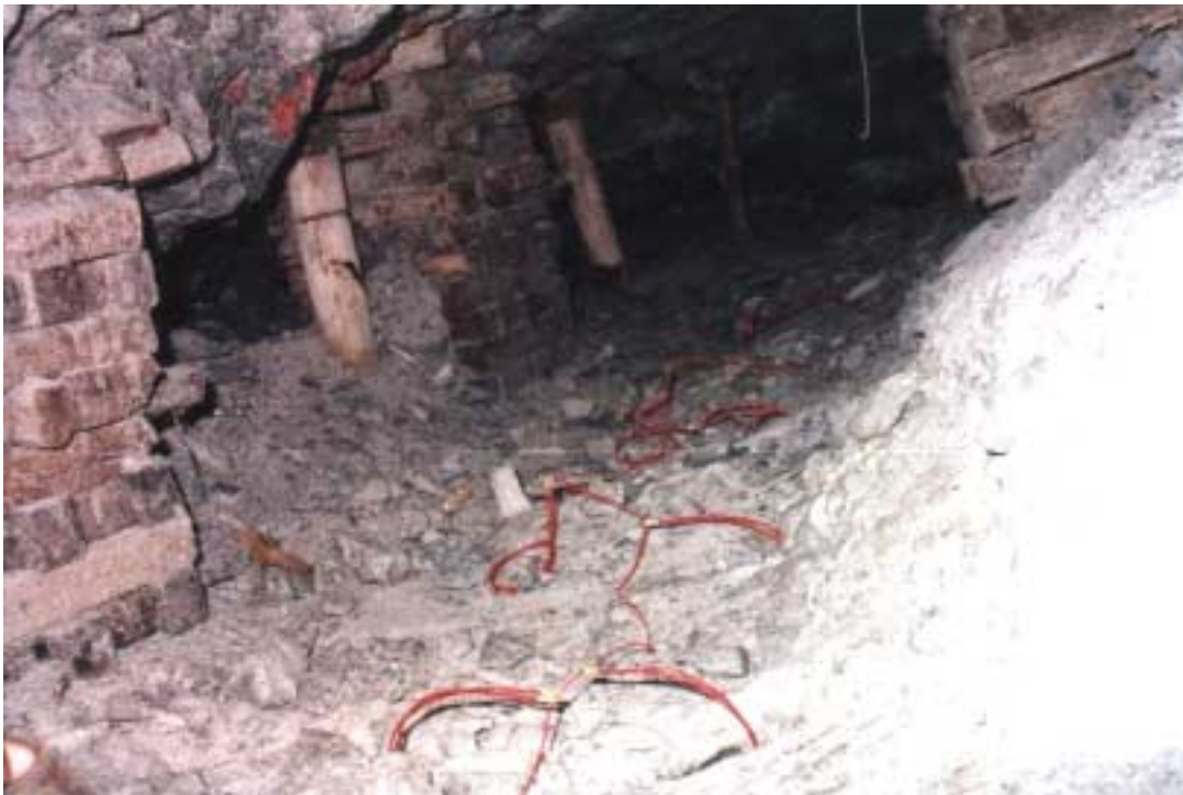
Figure 4.46 – Gully ripping blasting practice in a wide heading, which gives rise to conditions shown in Figure 4.45
