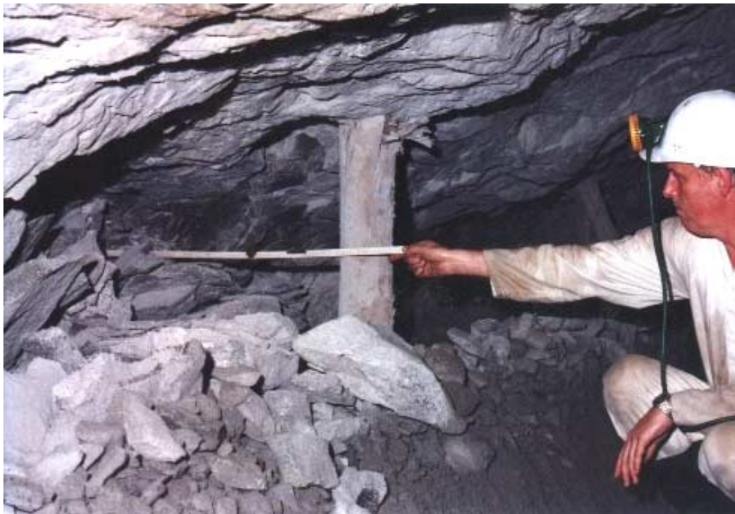
Figure 4.17 – Merensky Reef - lagging 1 m wide supported siding
