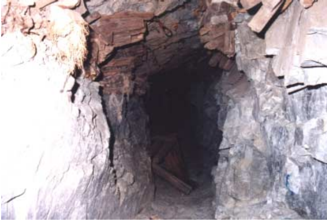
Figure 4.47 - VCR – good blasting practice - footwall lifted gully advanced incrementally by drilling horizontally in the gully face
