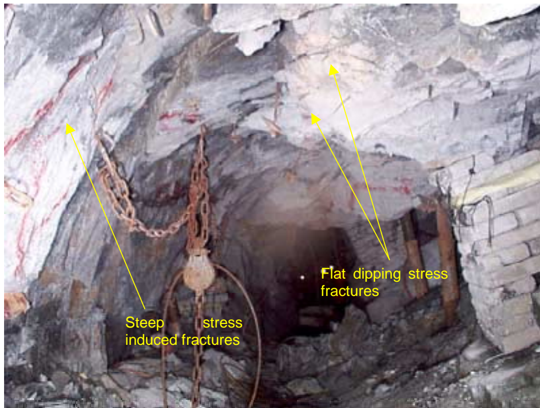
Figure 4.28 - Basal Reef - combined effect of an ASG heading, plus a lagging siding when strata is well bedded
