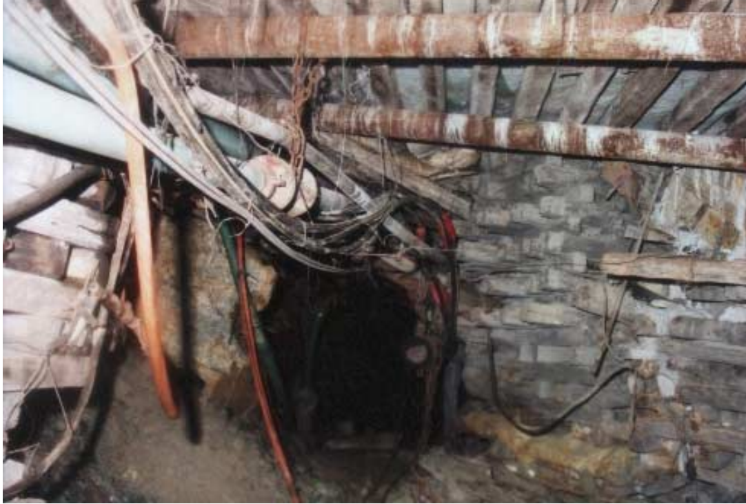
Figure 4.42 – Strike gully on the Carbon Leader reef at 2900 m depth, where a stable long term access has been achieved through using sets and void filling
