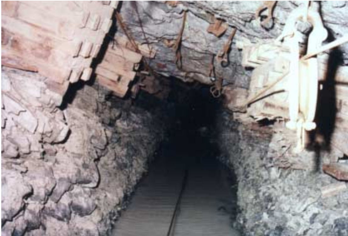
Figure 4.34 - Carbon Leader wide heading footwall lifted gully with good hangingwall conditions at 3200 m depth
