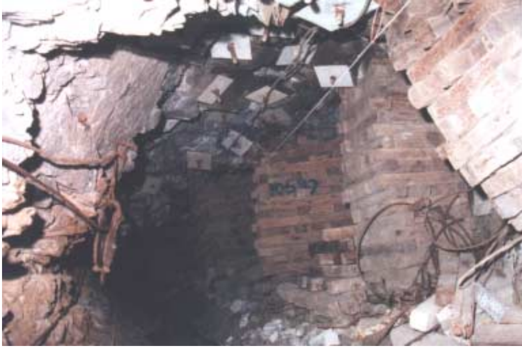
Figure 4.40 – Ground consolidation by injection grouting in the partially collapsed hangingwall of a VCR strike gully at 2800 m depth
