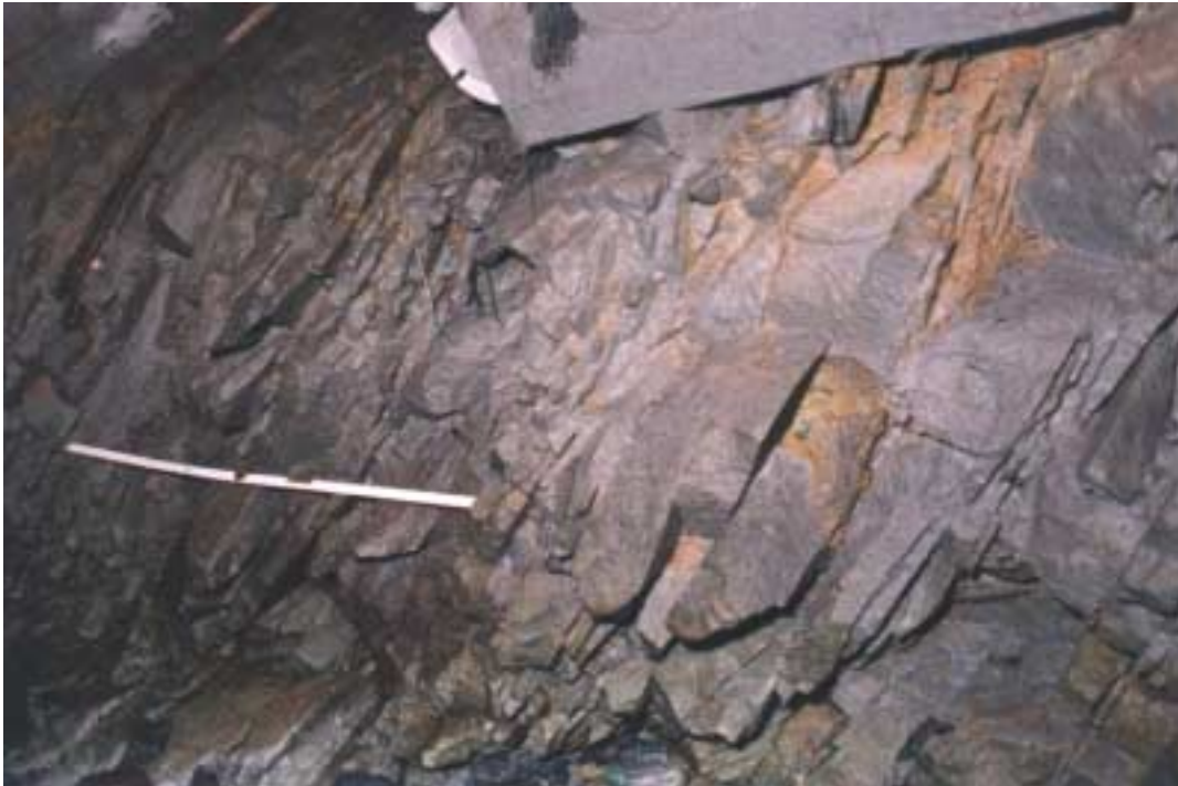
Figure 4.29 - Typical high density stress fracturing in gully sidewalls in VCR footwall quartzites
