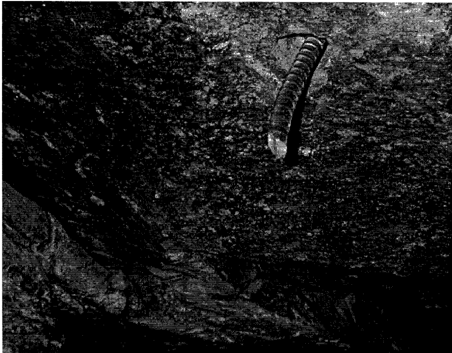
Photograph 3-4. Guillotining of hangingwall rock bolt.
