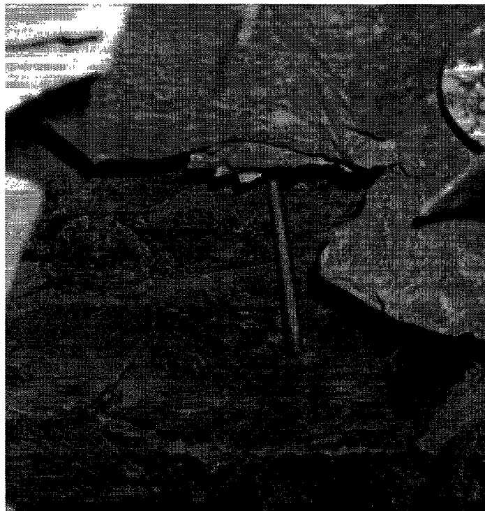
Photograph 3-5. Tensile failure of hangingwall rock bolt.
