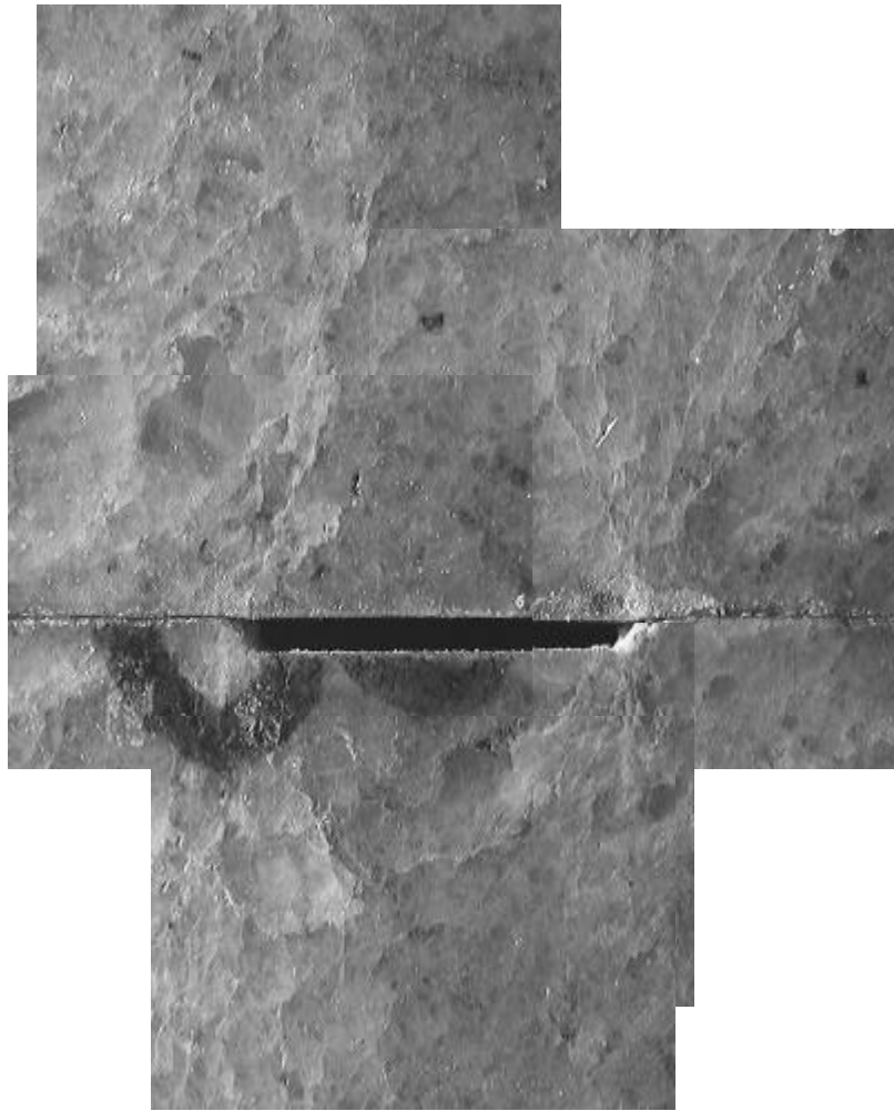
(a) Detail picture of fracturing around the narrow slot
