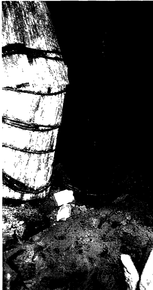
Figure 8.1.14 b) Loadmaster; note failure mechanism of foot of prop.
