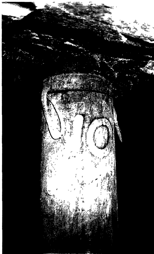
Figure 8.1.11 a) Turned Profile Prop, note brushing of prop top.
