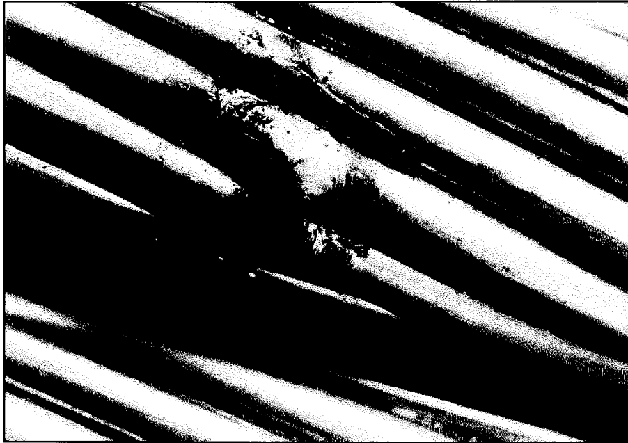
Figure 1: The photograph shows the weld damage on one of the specimens prior to testing
