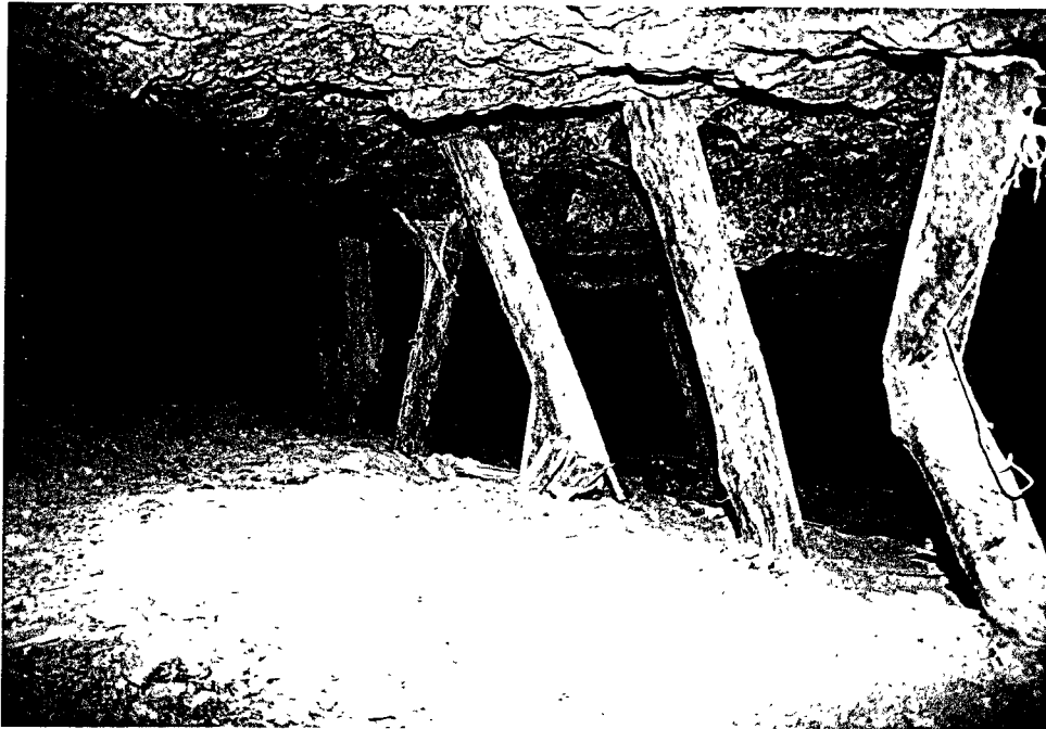
Photograph 7 : View of closure adjacent to pillar A in June 1994.
