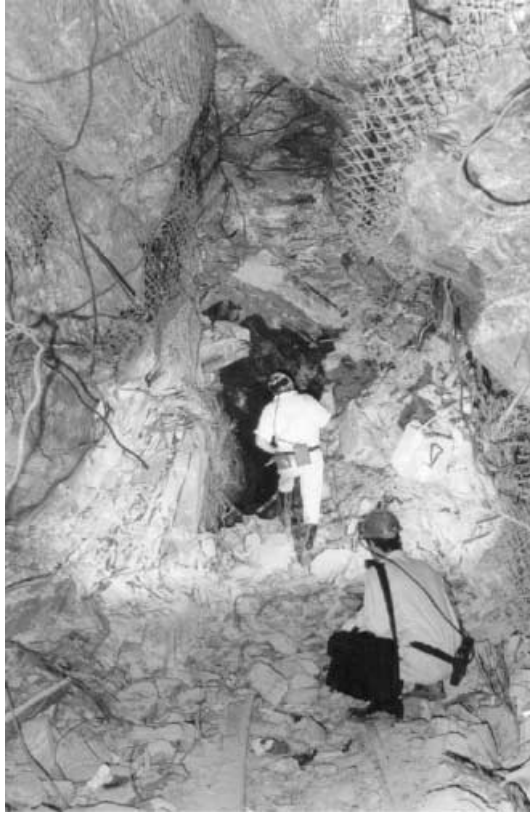
Fig. 1. Adverse haulage conditions at Hartbeestfontein Gold Mine in South Africa caused by slow time-dependent deformation processes in the rock. Note that this is not rockburst damage (courtesy W. D. Ortlepp)
