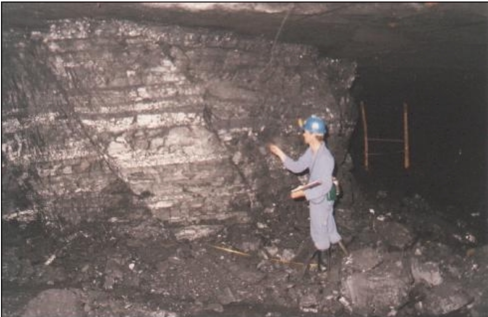
Figure 2-5 Major discontinuities in a pillar at the Piet Retief case study
