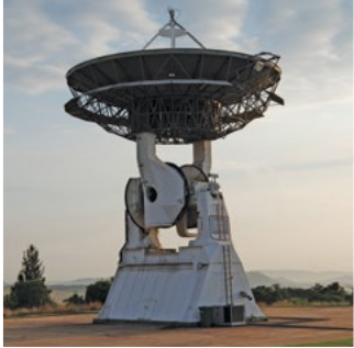
HBK-2: 12 m S- and ext C-band antenna with a 10°/sec slew rate, programme and auto-tracking. Installed in 1963 to undertake TOSS 3 and routine operations.
