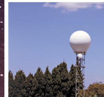
NOAA: 2.1 m L-band antenna, 2°/sec slew rate, programme tracking. Provides NOAA satellite reception.
