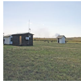
HMO: HBK hosts systems for SANSa Space Science, previously HMO, a national geomagnetic research facility and active participant in INTERMAGNET, which monitors the Earth's magnetic field
