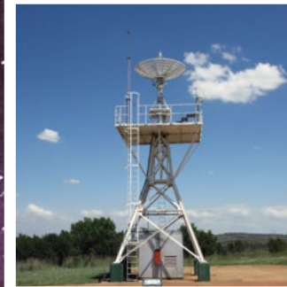
Modis: 3.2 m X-band antenna, 2°/sec slew rate; programme and step tracking. Provides Terra and Aqua satellite reception (2004).
