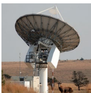
HBK-10: 11 m C-band antenna with a 5°/sec azimuth 5 slew rate, 1.4° elevation 6 , programme and auto-tracking. Installed in 2003 and used for housekeeping (maintenance) and TOSS.
