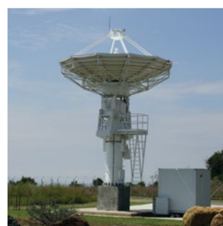
HBK-16: 7.3 m X-band antenna with a 3°/sec slew rate, programme and auto-tracking. Installed in 2008 to strengthen SAC's Earth observation capabilities.
