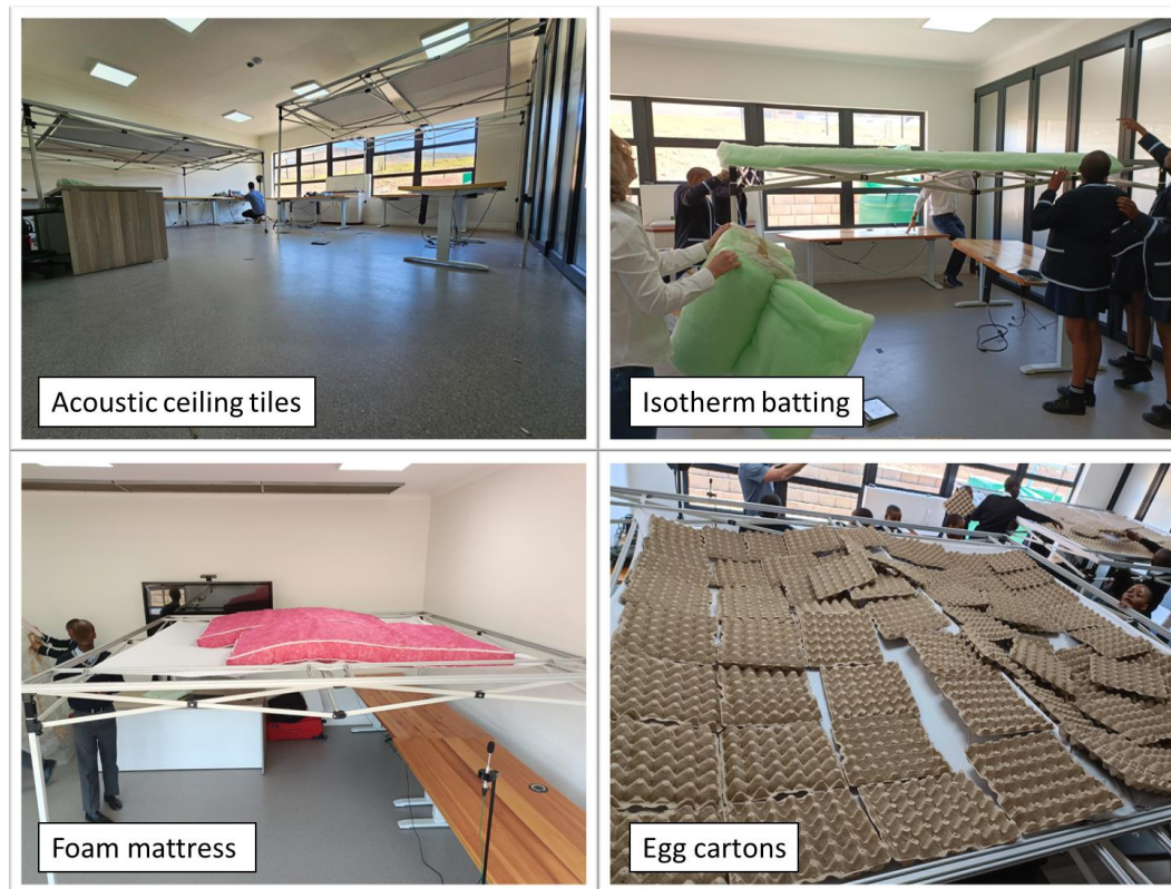
Figure 4. Photos of each intervention being installed.
