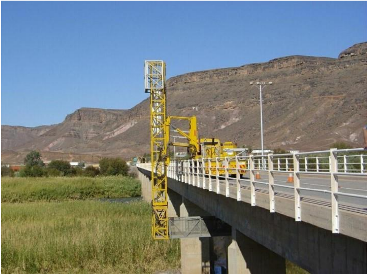
Figure 1-1: The Under Bridge Inspection Unit being used on the bridge across the Orange River at the Violsdrif border post between South Africa and Namibia (Source: SANRAL)
