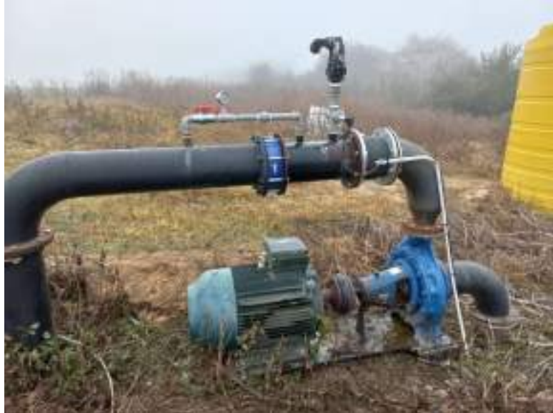
Figure 5: Controlled Pump and Pressure Sensor.
