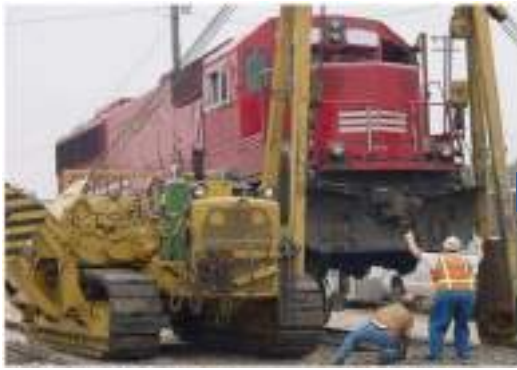
Figure 2: Locomotive Lifting process
