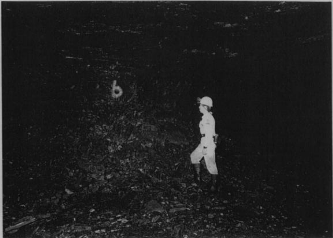
Figure 2.4. WIN (A) Rating 423 Poor. Pillar Scaling
