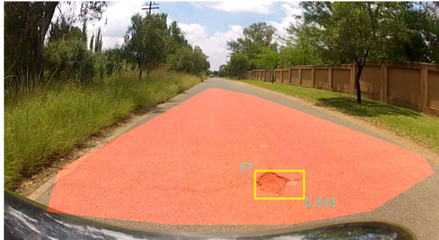
Fig. 8. Detection and size estimation of pothole
