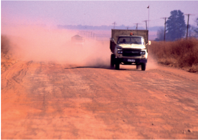
Fig. 1. An unsealed road constructed of weathered sandstone.
