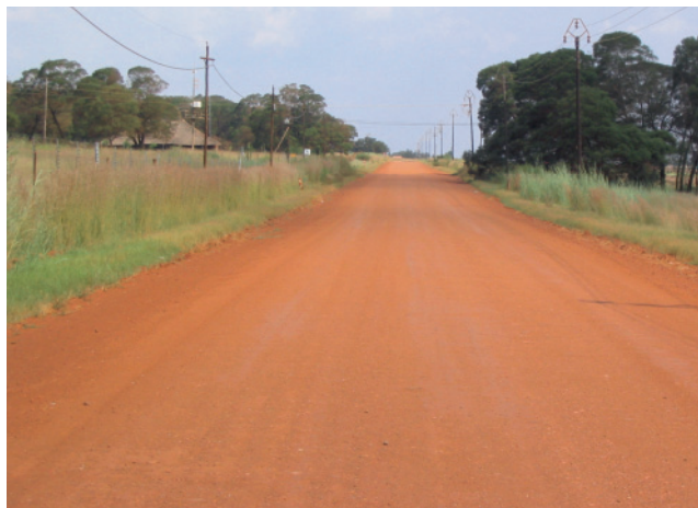
Fig. 3. Good unsealed road constructed from materials complying with the specification.
