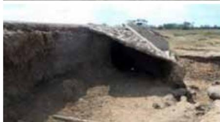
**Figure 5 Damage to culverts and erosion protection.**
