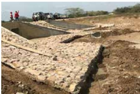
**Figure 13 Construction of culverts and erosion protection works.**
