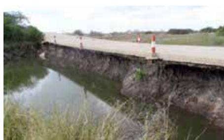
**Figure 3 Erosion and undercutting of concrete fords.**
