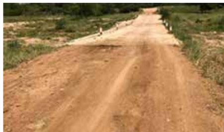
**Figure 4 Damage to the road approaching concrete fords.**
