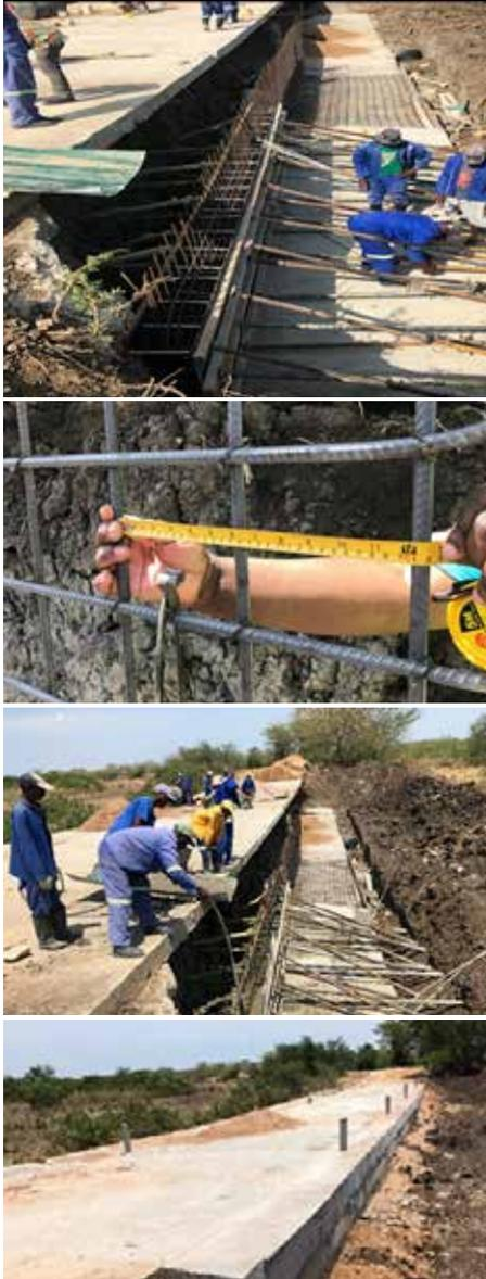
Figure 10 Construction of concrete wall.
