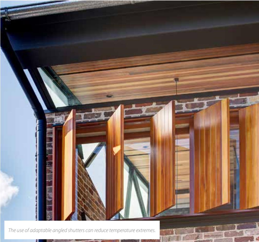
*The use of adaptable angled shutters can reduce temperature extremes.*
