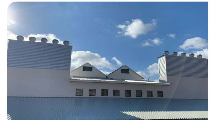
Above: Solar chimneys, a natural ventilation strategy.
