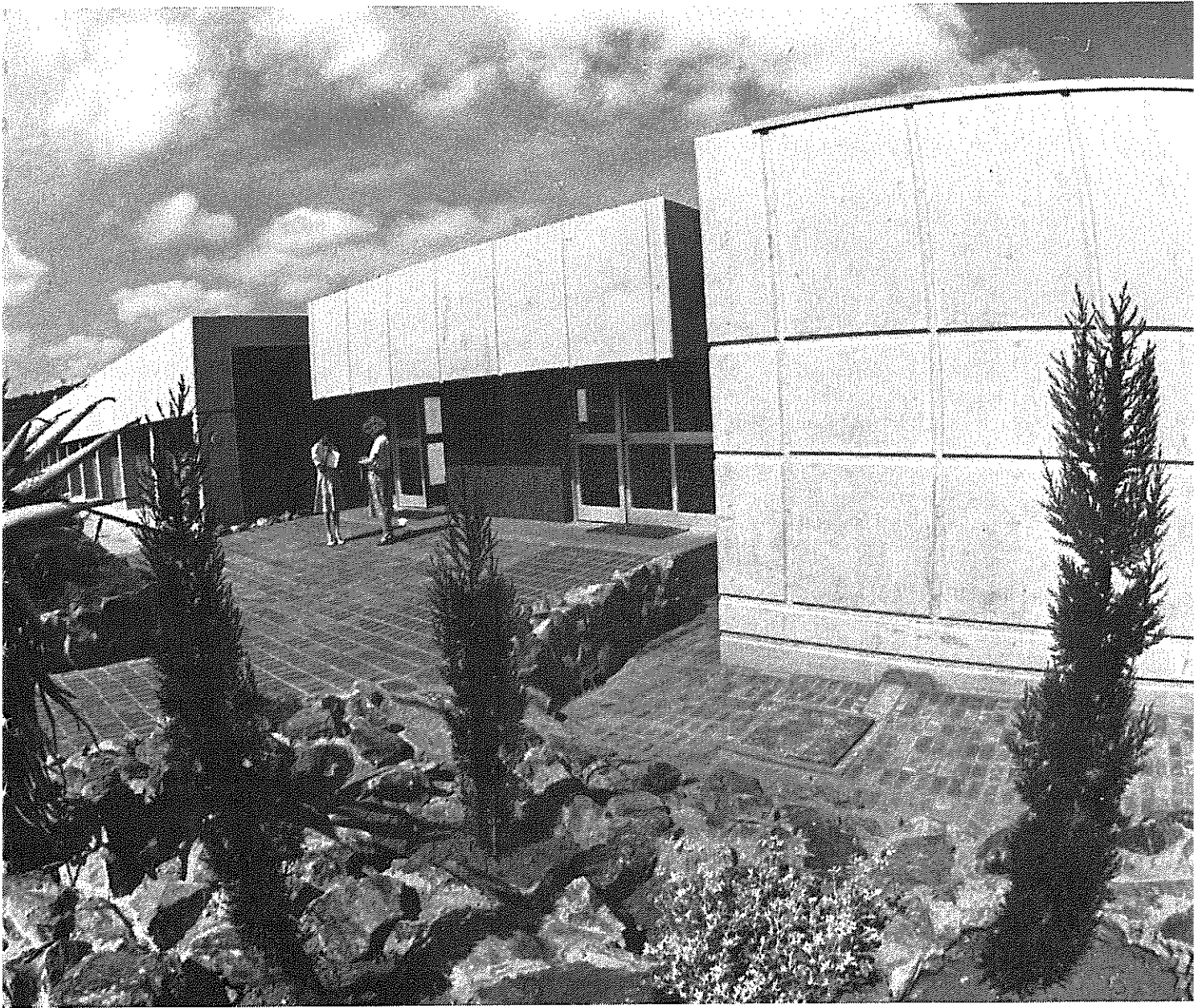
A view of the Computing Centre building.
