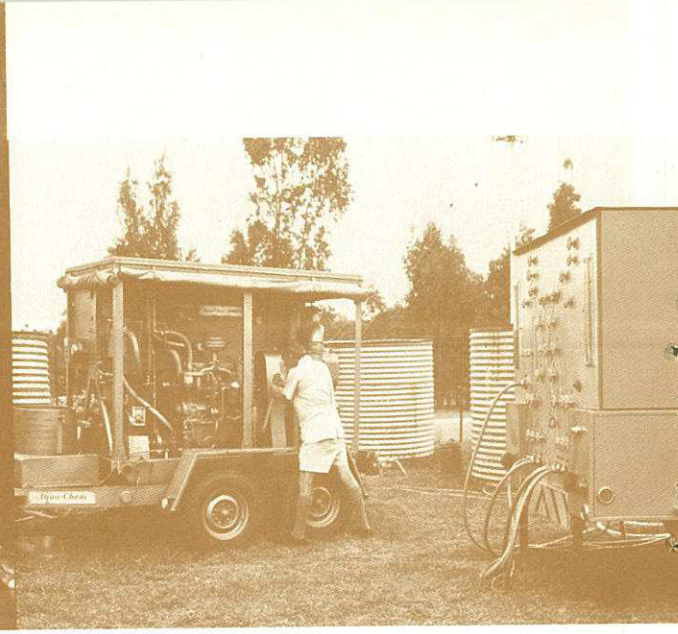
A vapour compression evaporation unit with ion exchange pretreatment unit.
