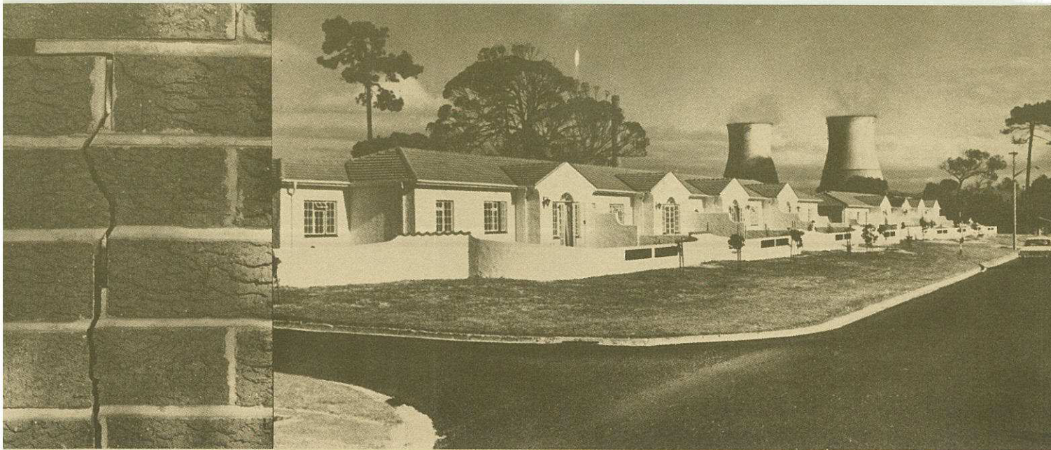
An example of the serious damage moisture expansion can cause in clay brickwork.
