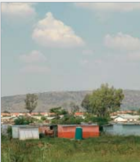
The CSIR provides knowledge-intensive solutions to support all spheres of government in managing housing development
