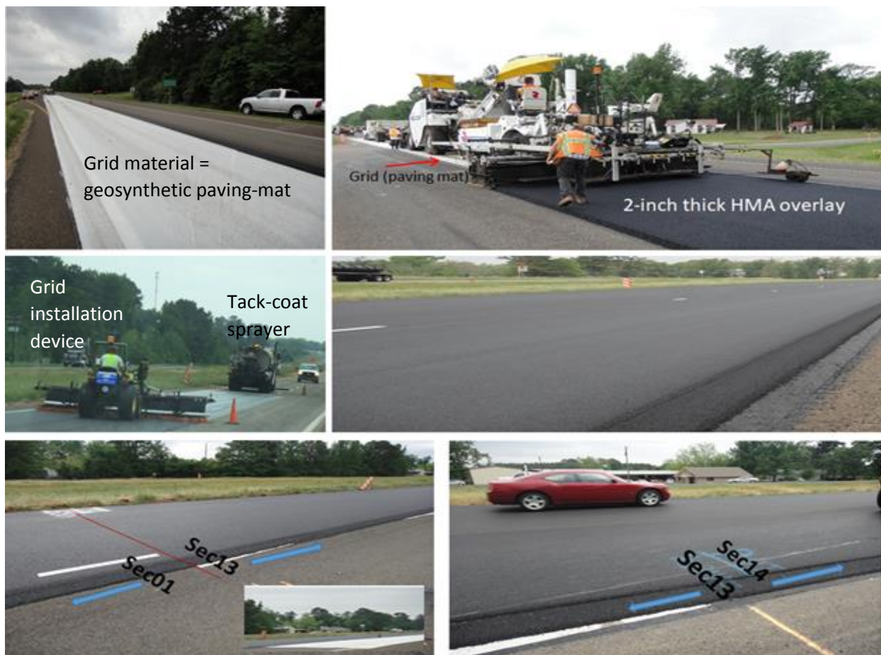
15 16 Fig. 4. Geosynthetic Installation and HMA Overlay Construction.
