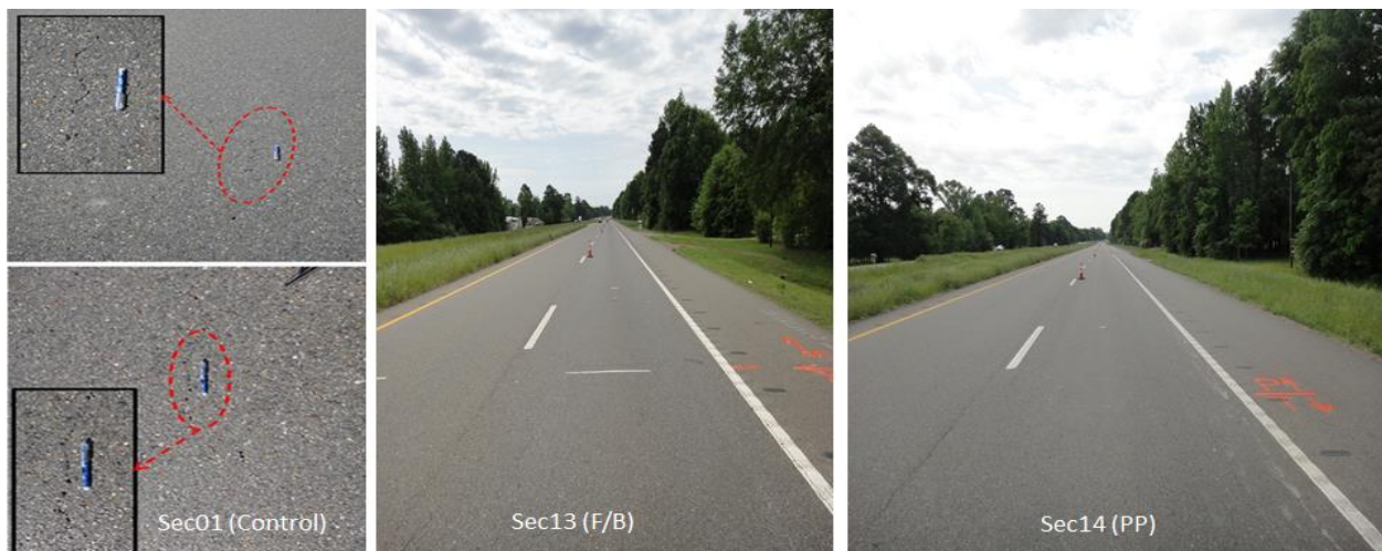
26 27 Fig. 11. Pictorial Surface View of the US 59 Test Sections.
