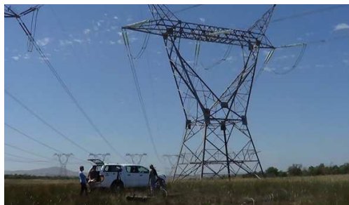
Figure 7: KIPTS insulator testing station [2]
