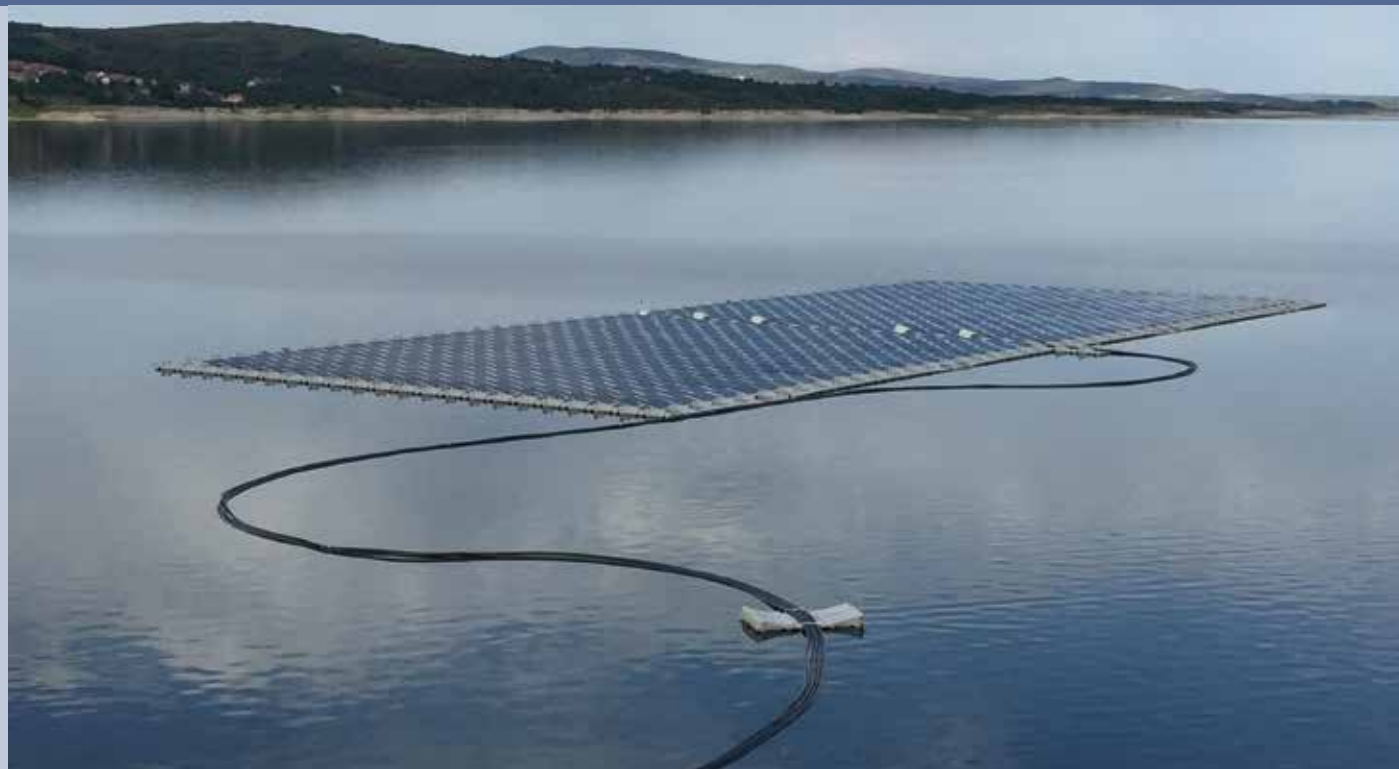
Fig. 1 - 220 kW PV floating system in the North of Portugal (Photo: LNEG).
