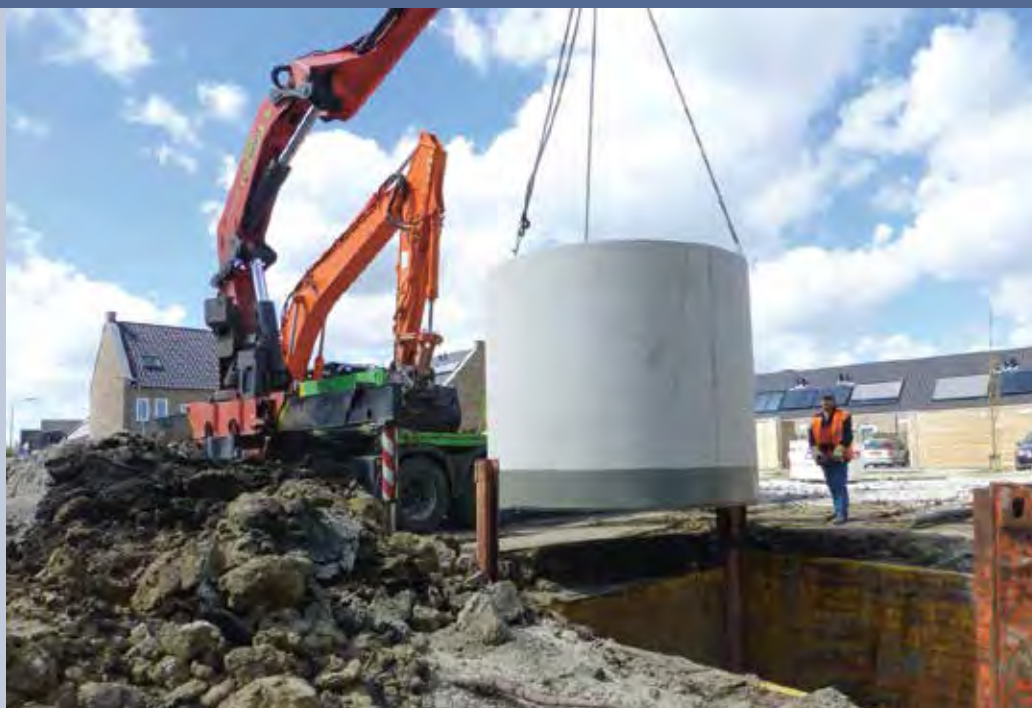
Fig. 2 - Installation of ice/water storage tank Goes, Province Zeeland, courtesy of Marsaki (Photo: Marsaki & RWS partner in wonen).
