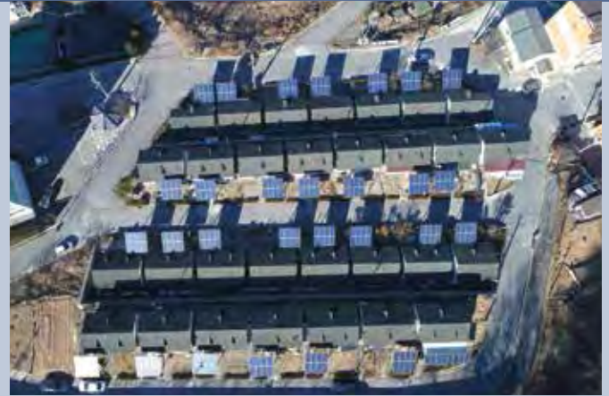
Fig. 2 - Combined PV and solar thermal system, Samcheok-si, Gangwon-do, Korea.
