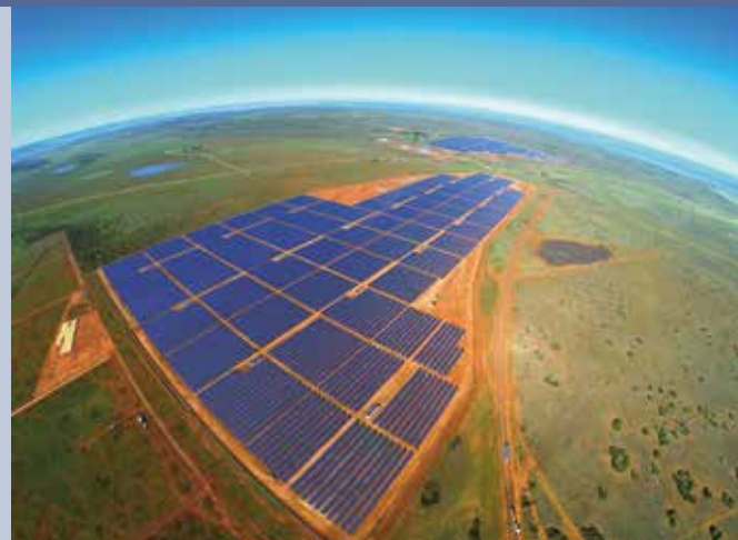
Fig. 5 – 75 MW PV plant built by COBRA in Kimberley, Rep. of South Africa (Photo: ©Grupo Cobra).
