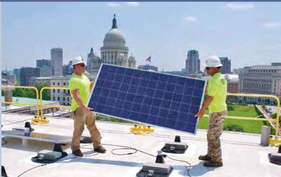
Fig. 2 - Phil Doucette (left) and Jim Mitchell (right) of Newport Renewables install solar panels on the Powers Building, part of a 330 000 kWh, 890 panel project covering three government buildings in the Capitol Hill complex. The Rhode Island Statehouse is visible in the background (Photo: Robert Beadle).
