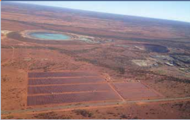
Fig. 3 - The DeGrussa Solar Farm. The DeGrussa Solar Project was successfully commissioned at Sandfire's DeGrussa Copper-Gold Mine. It has 34 080 solar PV panels with a single-axis tracking system mounted on 4 700 steel posts.
