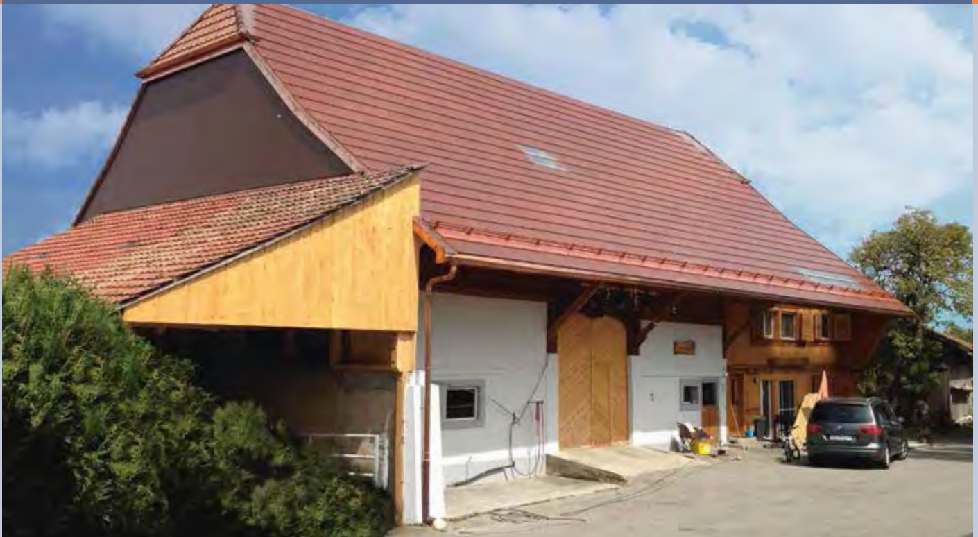
Fig. 2 - A southwest view of the PV installation on a farm house in Ecuivillers, Fribourg, Switzerland. With their terracotta appearance, these innovative PV roof tiles provide a perfect integration into the townscape (photos: © CSEM & © ISSOL).
