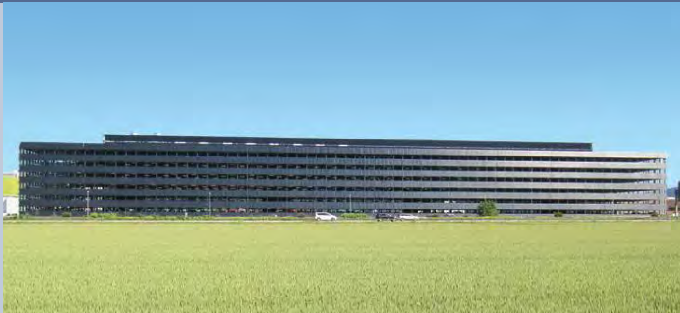
Fig. 1 - Swissolar Prize Winner 2017: The most powerful PV façade in Switzerland on the F. Hoffmann-La Roche AG's parking garage in Kaiseraugst, Switzerland. This façade system has a total installed capacity of 633 kWp and an estimated production of 473 000 kWh per year (Photo: © BE Netz AG, Ebikon).
