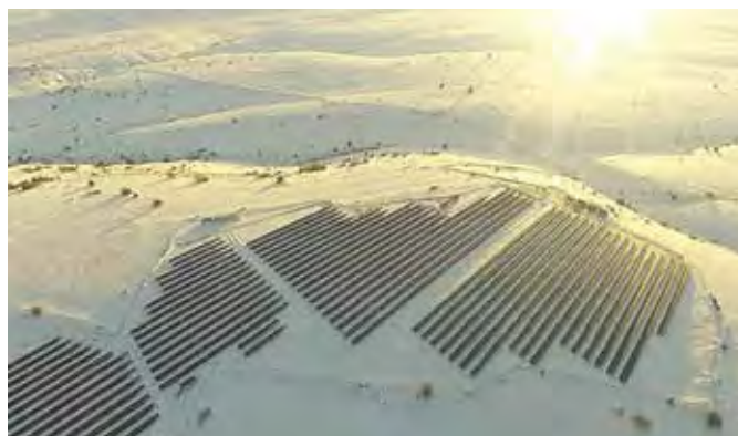
Fig. 1 - One of the PV power plants in Kayseri (12 MW) [17].
