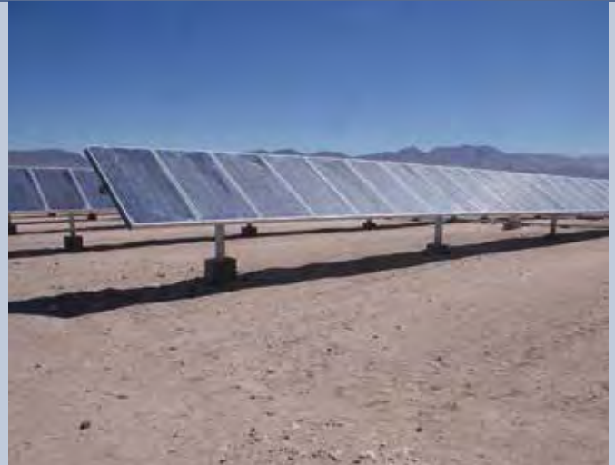
Fig. 2 - Calama Solar 3. The excellent local radiation conditions, in combination with the one-axis tracking systems, makes this 1 MW plant to deliver an outstanding annual generation of 2900 MWh (data April 2012 - March 2013).
