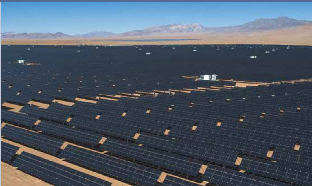
Fig. 3 - Large PV Plant. 141 MW Luz del Norte PV Plant (First Solar) located at Copiapó, Atacama Region, Chile.
