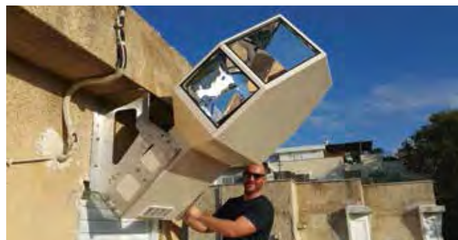
Fig. 2 - Solight installing its lighting system.
