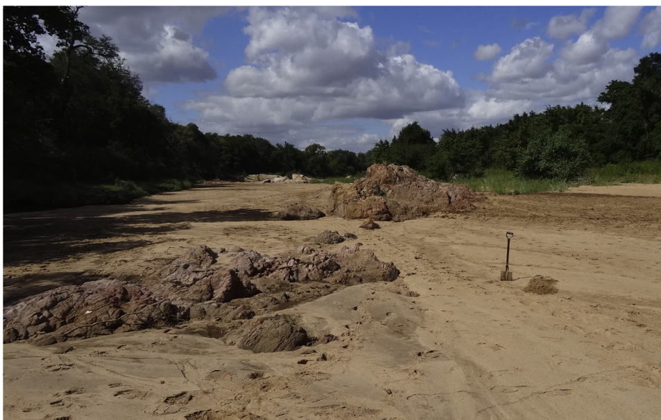
Fig. 7. In-channel outcrops at chainage 1200 m that almost block the sand river.
