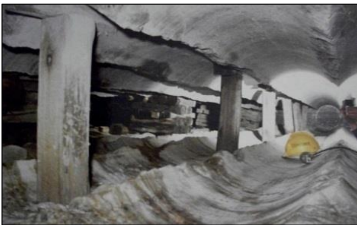
Figure 1. The completed slot bored by sequential raisebore holes
