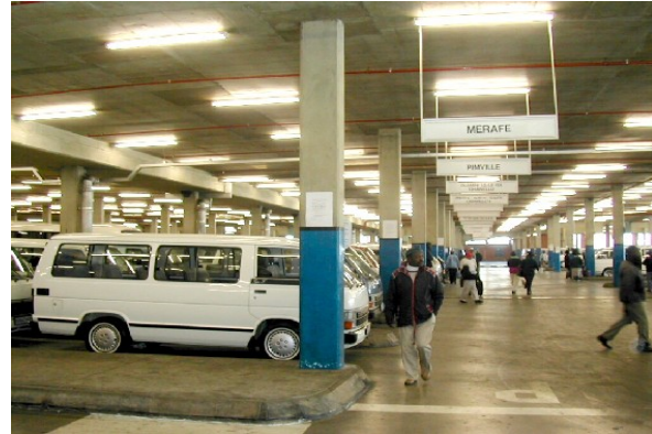
Figure 10: Efficient lighting and signage contribute to reducing congestion and increasing levels of safety.
