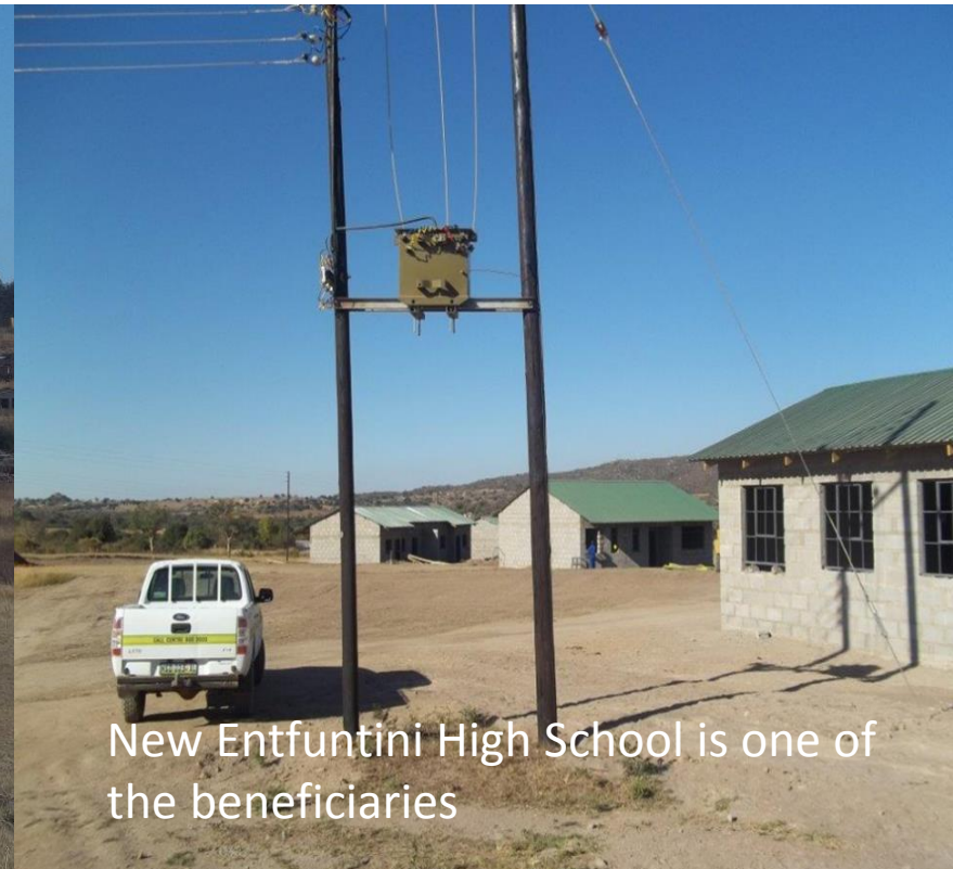
43 homesteads were electrified under this group scheme at Lushikishini
