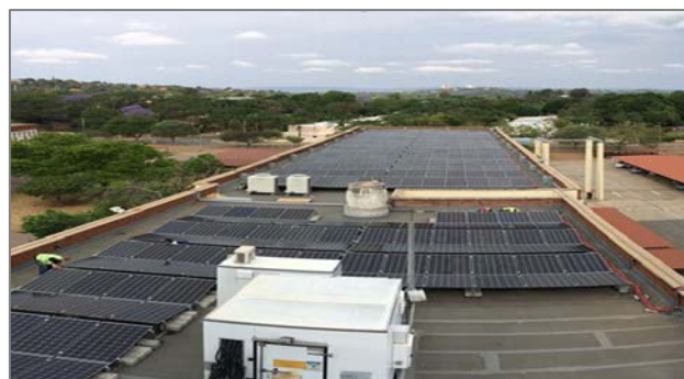
Picture 3: CSIR's of 250 kWp west facing rooftop plant
